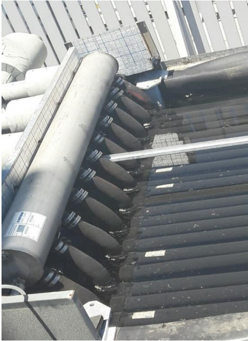
Repair of Ice banks by FAFCO (Switzerland)
