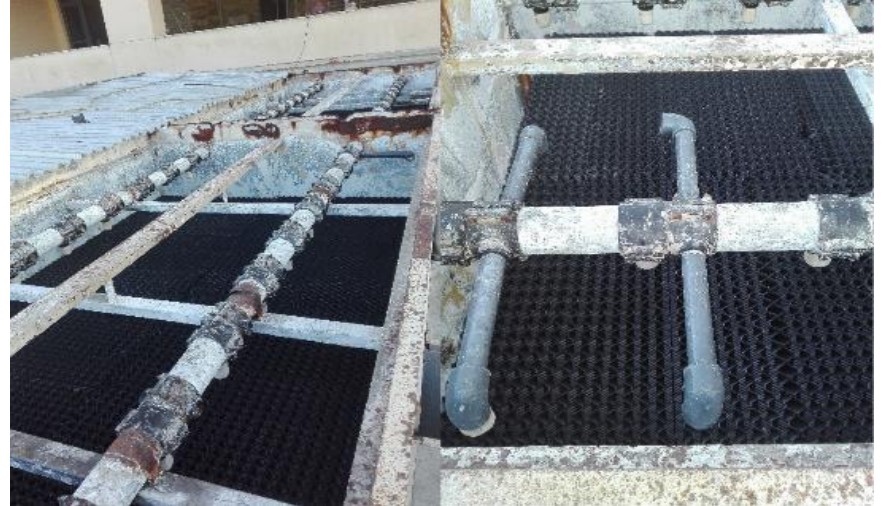
Chemical Cleaning of Cooling Towers
