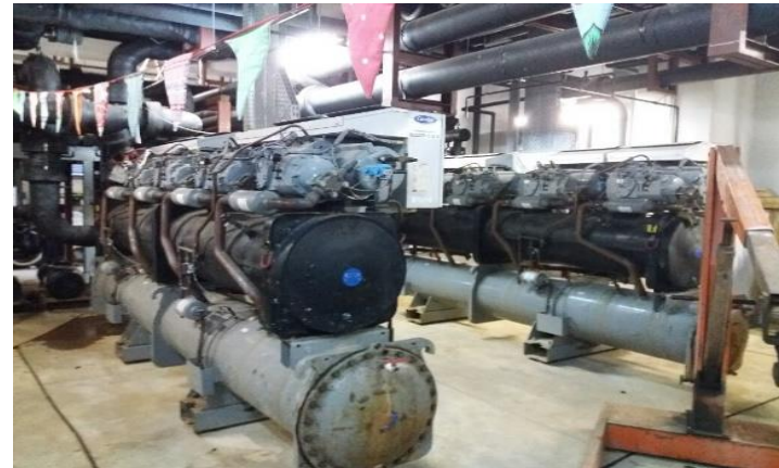
Carrier - Chiller repair and maintenance
