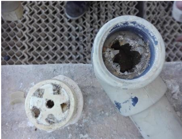
Water Softener Repair
